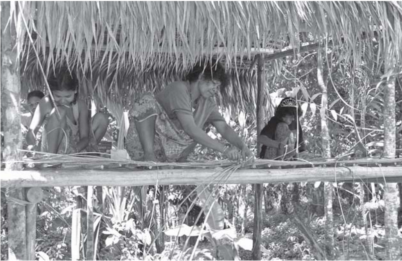
Plate 5.5 Chewong women at Kuala Gandah working on the flooring of a new house during the house-building season in early 2005. (Anja Lillegraven)
