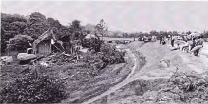
Plate 43. Demolition of Orang Asli house at Bukit Lanjan (Damansara Perdana, Selangor). In a deal aided by the JHEOA, the Orang Asli reserve at Bukit Lanjan was transferred to the Emkay Group for well below its market value. Part of this land was then (re)acquired by the government for the construction of the Damansara-Puchong Highway – at market value. Then, in a move designed to demonstrate the might and power of the players in the development vision of the nation, two Orang Asli houses were summarily demolished. No proper notice was given to the occupants. Neither was their plea for a short postponement (to move their belongings to alternative housing) entertained. (CN-1998)
